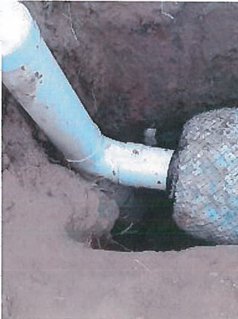
CORRECTED SWEEP ON INSPECTION POINT
