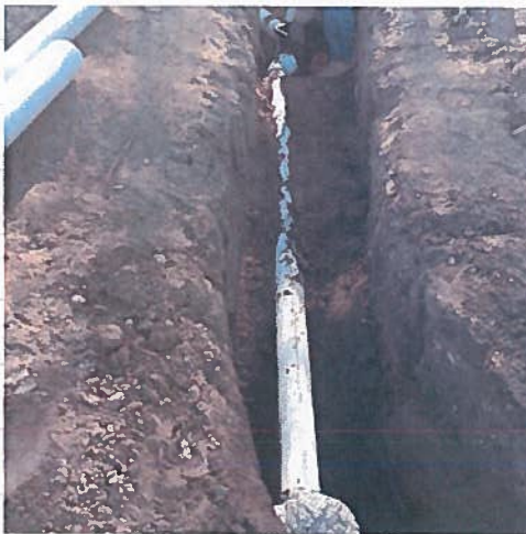
PIPING LEADING FROM D-BOX TO DISPOSAL FIELD
