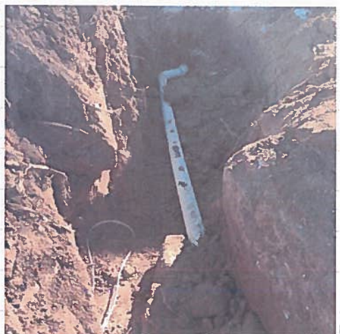
PIPING LEADING FROM D-BOX TO DISPOSAL FIELD
