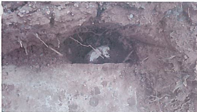
EXPOSED INLET PIPE: SIDE ENTRY
